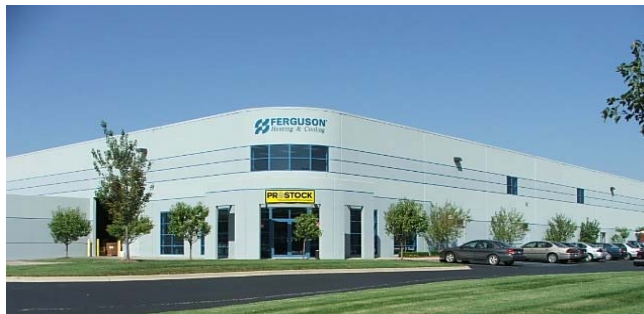
Ferguson Enterprises (HVAC)
