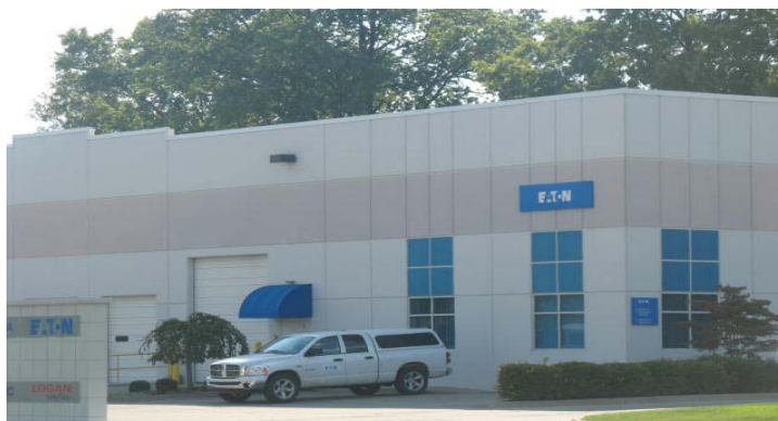
Eaton Electrical Logan Fabricom
